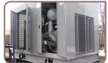
Electric Generator - Diesel Fueled
